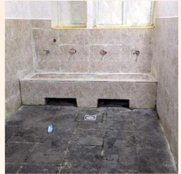
Gondar Hospital toilet block renovation, completed January 2024
